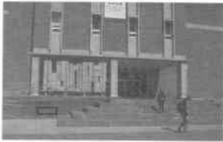
Figure 2. The Administration Building
